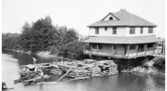
"Superintendent Burton Deane's house being moved to the east side of the Elbow River.", 1929-08, (CU193485) by Oliver, W. J. Courtesy of Glenbow Library and Archives Collection, Libraries and Cultural Resources Digital Collections, University of Calgary. https://digitalcollections.ucalgary.ca/asset-management/2R3BF1O1WDUK .
