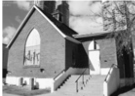
Westbourne Church in April, just prior to its demolition in June 2017. Calgary Heritage Initiative.
