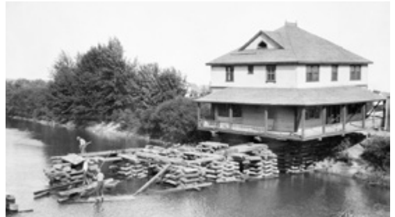
"Superintendent Burton Deane's house being moved to the east side of the Elbow River," 1929-08, (CU193485) by Oliver, W. J. Courtesy of Glenbow Library and Archives Collection, Libraries and Cultural Resources Digital Collections, University of Calgary. https://digitalcollections.ucalgary.ca/asset-management/2R3BF10WDUK .
