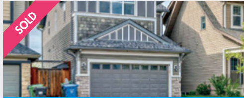
265 AUBURN GLEN MANOR SE ~ $835,000
