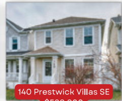
140 Prestwick Villas SE $529,900
