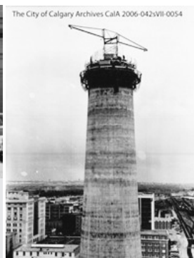
Husky Tower over 200 feet in height - 27 feet of concrete poured a day, City of Calgary Archives, item CaIA 2006-042sVII-0054.
