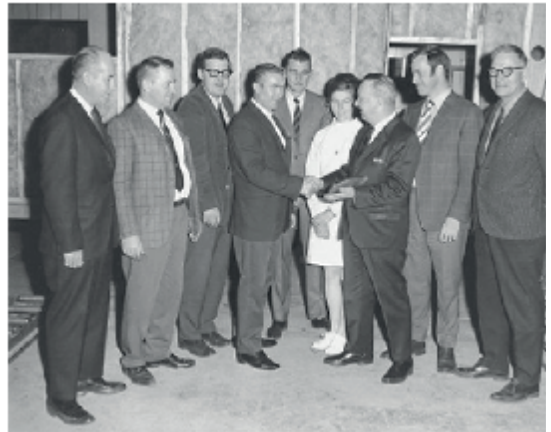
ATCO Manager presenting Safety Performance Awards to the Construction Division
