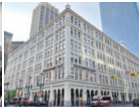
Hudson's Bay Company building, corner of 1 St SW and 8 Ave, 2019. Photo courtesy of Olivia Breytenbach, Calgary Heritage Initiative.
