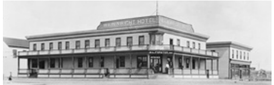
"Wainwright Hotel, Wainwright, Alberta.", [ca. 1911-1912], (CU1126598) by Unknown. Courtesy of Glenbow Library and Archives Collection, Libraries and Cultural Resources Digital Collections, University of Calgary. The hotel burned down in 1929. A reconstruction is in Heritage Park, Calgary, Alberta. https://digitalcollections.ucalgary.ca/asset-management/2R3BF1FJKK33?WS=SearchResults .
