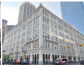
Hudson's Bay Company building, corner of 1 St SW and 8 Ave, 2019. Photo courtesy of Olivia Breytanbach, Calgary Heritage Initiative.
